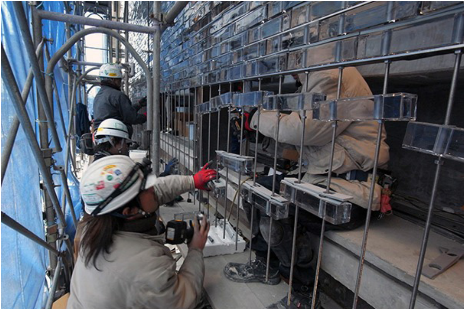
The blocks are assembled on-site, using stainless steel bolts and bars for structural integrity.
